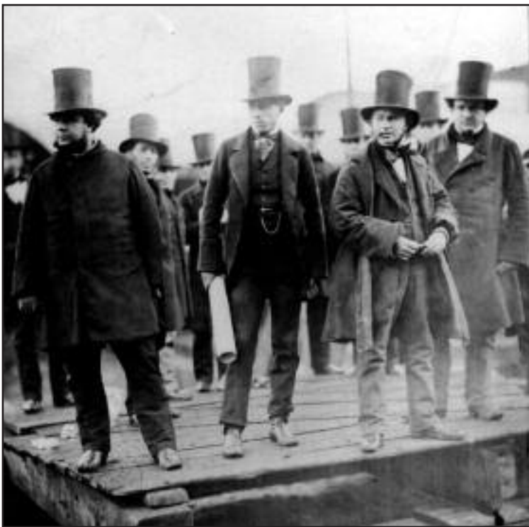
This page (clockwise from above), launch day of Brunel's ill-starred leviathan, SS 'Great Eastern', 1857. Brunel (second from right), watches the ship take to water with its Master, William Harrison (far right); the acclaimed, wealthy engineer at 51, painted by John Callcott Horsley; his office; one of the original Brunel 'broad gauge' locomotive rails, used as a safety barrier at Neyland, Pembrokeshire; the SS 'Great Eastern', built at Millwall, was nearly 700ft long and weighed just under 19,000 tons. It was broken up in 1888/89
